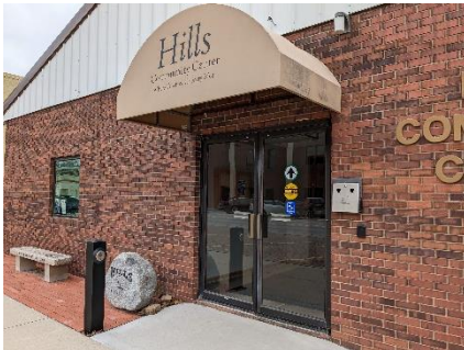
Hills Community Center, 110 E Main St
