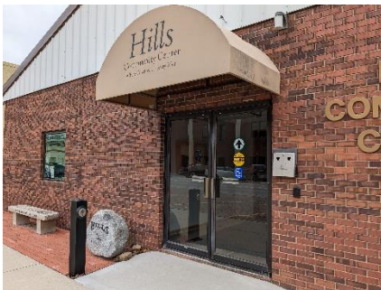
Hills Community Center, 110 E Main St
